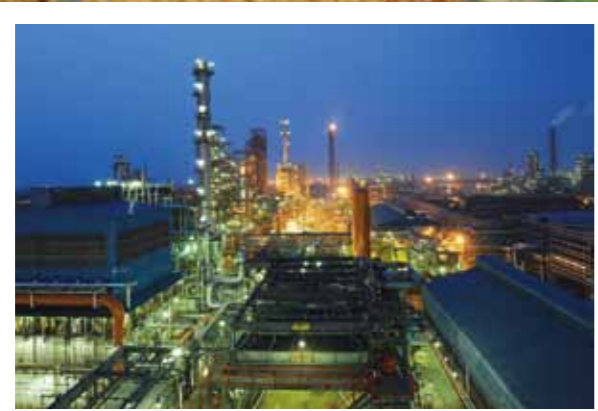
Hydrocracker and Hydrogen Generation Project, Haldia Refinery, India.
